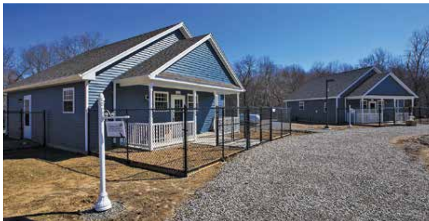
The two new canine cottages.
